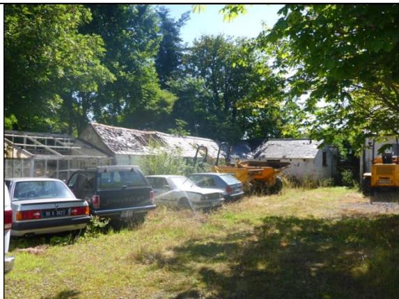
Plate 4.25 Outbuildings and rear gateway in eastern corner of courtyard, Clay Farm
